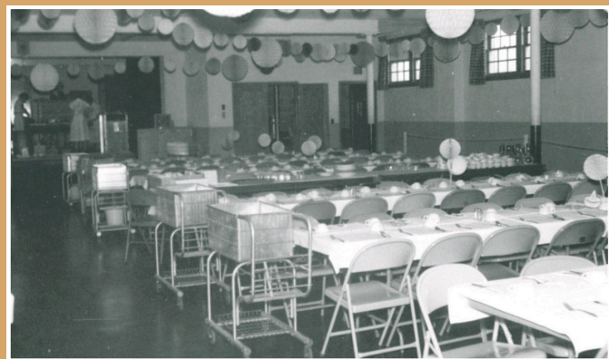
Church hall (basement of building)
