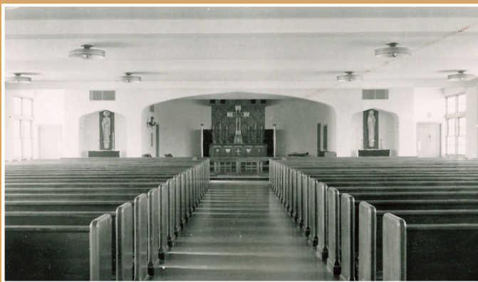
Church naïve (second floor of building)
